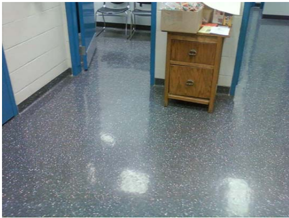
EPIC (predecessor) – after 4 years, sheet vinyl in main lobby of pet clinic
